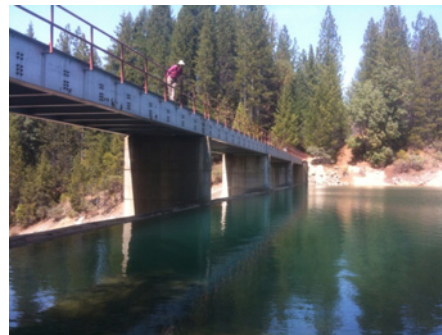
Scotts Flat spillway, March 27, 2010
