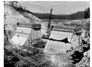
Building Scotts Flat Dam, 1964 (NID website)
